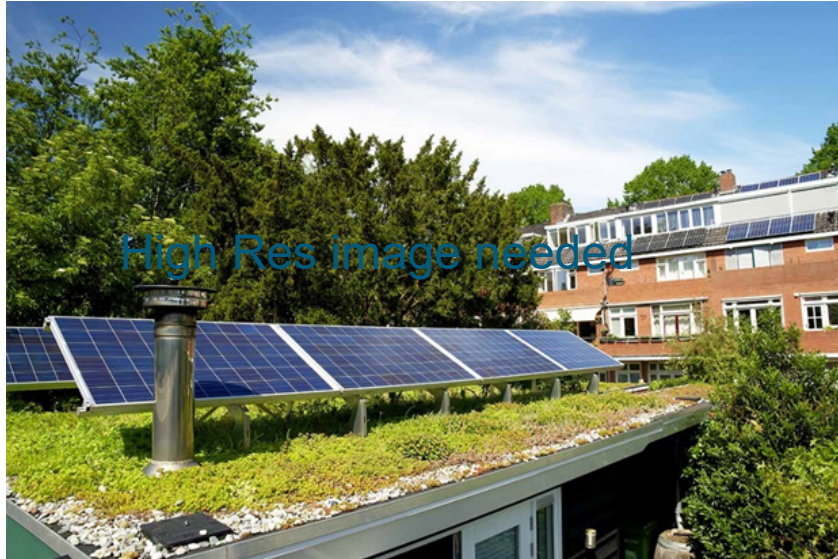
Figure 5: Example of a biosolar roof
